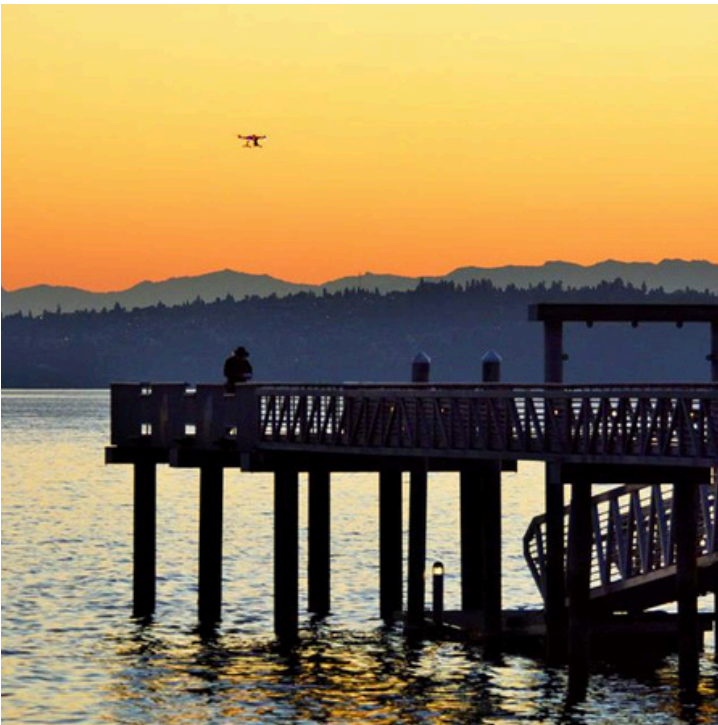
Photo of Harper Pier
