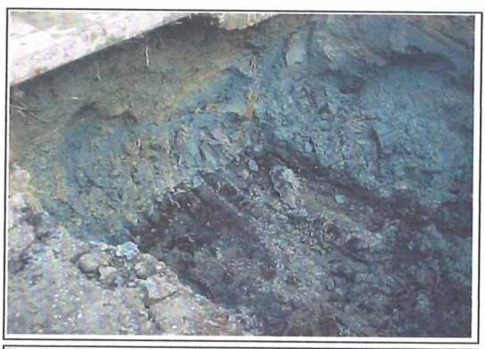
Photo 6. Soil excavation in former tank pit. Brown peat layer visible in bottom.
