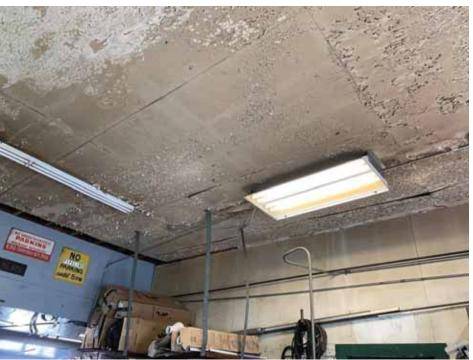
**Photo 42:** Subject Site – View showing evidence of water damage on the ceiling over the workshop.
