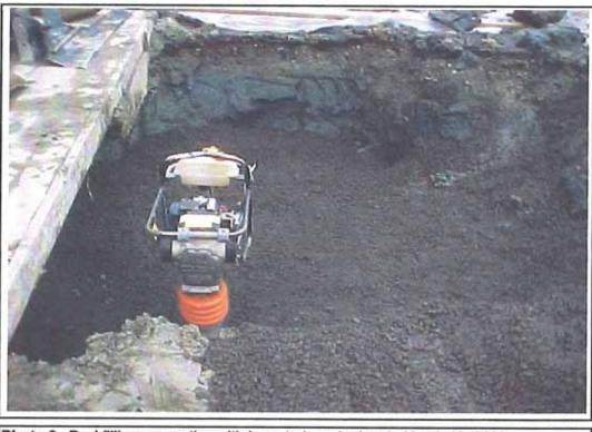
Photo 8. Backfilling excavation with imported crushed rock, March 13, 2002.
