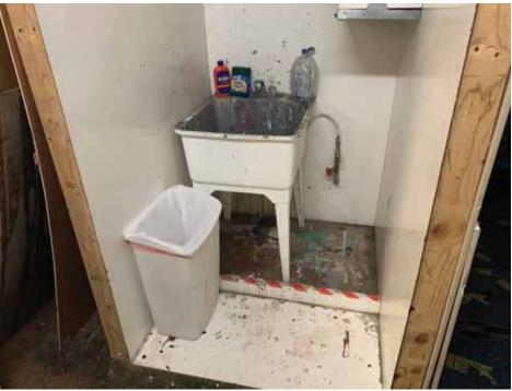
**Photo 18:** Subject Site – View showing sink with floor drain in the backstage area. No oil staining or sheen observe.
